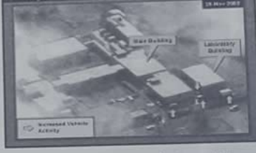
Pre-Inspection Material Removal Amiriyah Serum and Vaccine Institute
